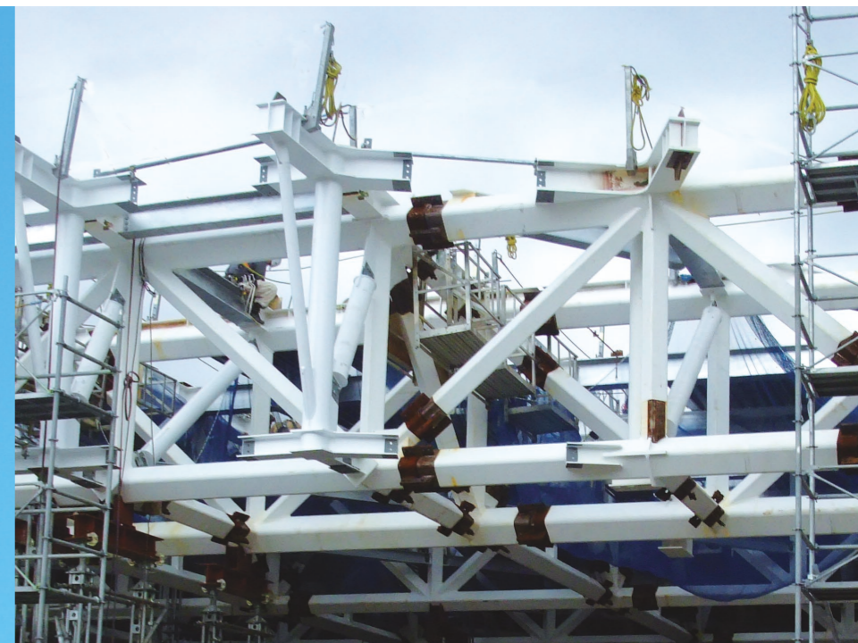
Steel Structure Roof (Square Hollow Section)
